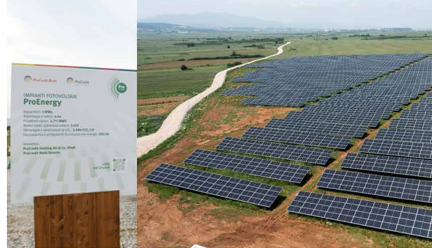
PARKU SOLAR PROENERGY 3MW
