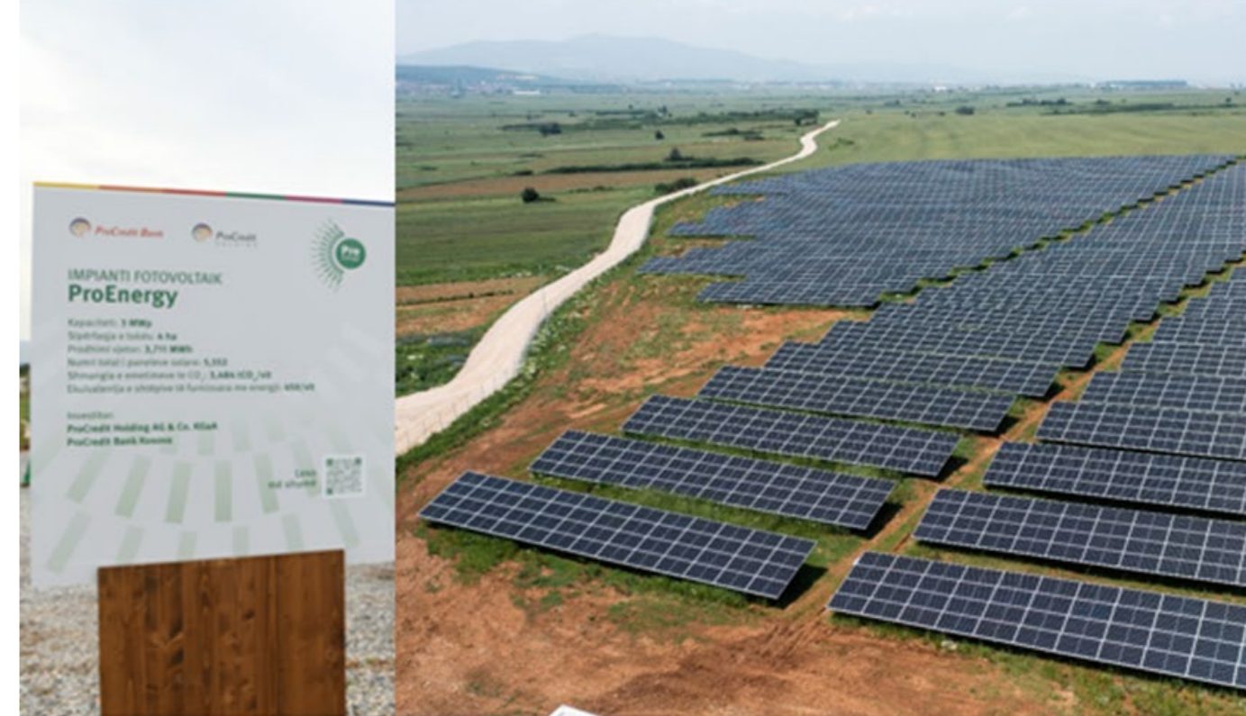
PROENERGY 3MW SOLAR PARK
